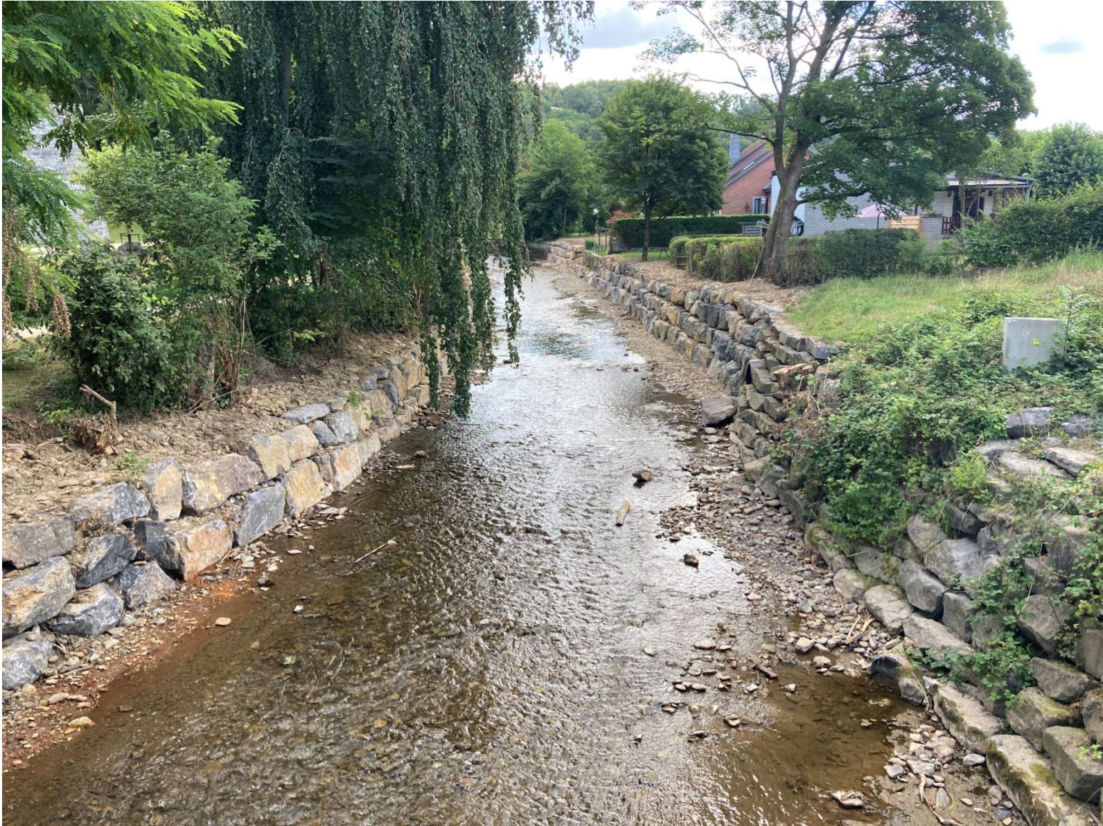
Aisne - bank riprap with parallel-faced blocks
